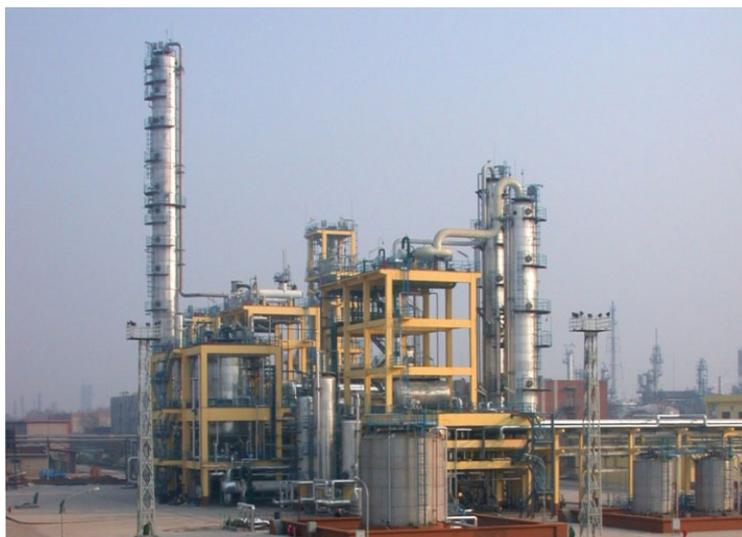
Fig. 2 2-Ethylhexanol plant built by Sinopec Qilu Petrochemical Co. Ltd., China, employing the LP Oxo<sup>SM</sup> Process
