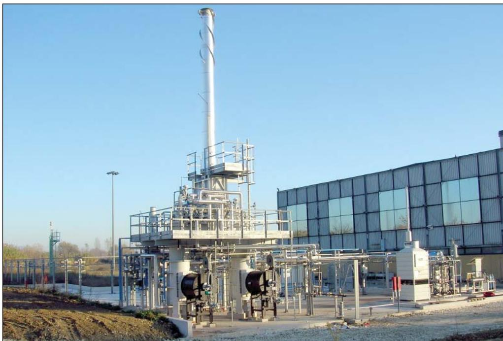
Fig. 1. Membrane reforming reactor for hydrogen production (20 Nm<sup>3</sup> h<sup>-1</sup>) in Chieti Scalo, Italy (Courtesy of Tecnimont KT SpA, Italy)
