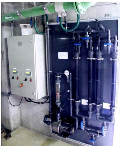
Fig. 4 Hypocell<sup>®</sup> B4 electrochemical disinfection device (G.E.R.U.S. mbH, Germany), with four pipe reactors equipped with mixed iridium/ruthenium oxide-coated titanium electrodes in a cooling water system, installed at a German paper mill
