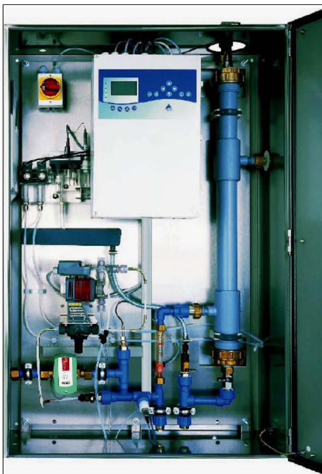
*Fig. 3 Electrochemical disinfection device AQUADES-EL (AquaRotter GmbH and G.E.R.U.S mbH, Germany) equipped with mixed iridium/ruthenium oxide-coated titanium electrodes: right-hand side: reactor pipe with inserted electrode stack; upper middle: power supply and control unit; upper left: amperometric free chlorine sensor equipment*
