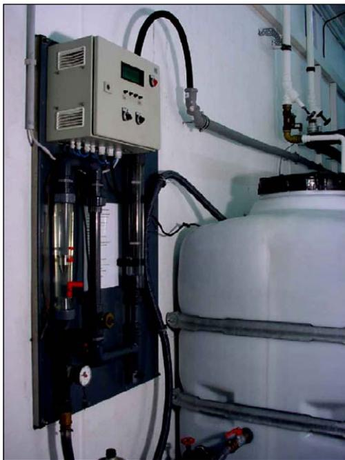
Fig. 6 Hypocell<sup>®</sup> B4 electrochemical disinfection device (G.E.R.U.S. mbH, Germany) equipped with platinised titanium electrodes, mounted in a car wash station
