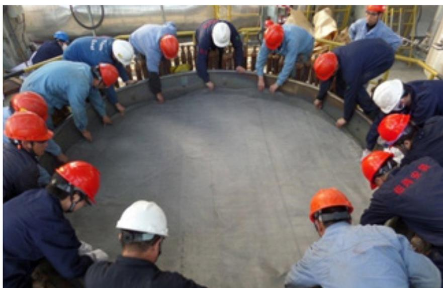
Fig. 4. Installation of a gauze pack at a customer plant supplied by Paite, Johnson Matthey's Chinese licensee
