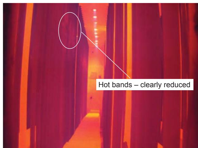
Fig. 5. Tube appearance two months after the carbon incident, illustrating some improvement
