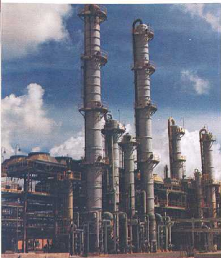
Butyraldehyde plant employing low-pressure oxo process at Ponce, Puerto Rico, started up extremely smoothly during early 1976. Figs. 2 and 3
