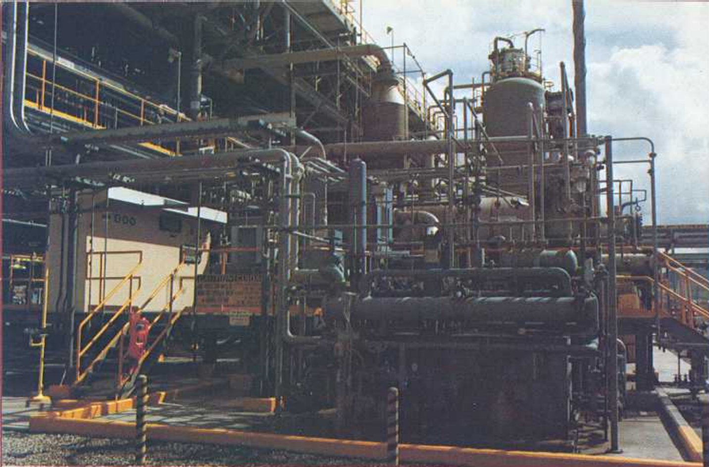
Butyraldehyde plant employing low-pressure oxo process at Ponce, Puerto Rico, started up extremely smoothly during early 1976. Figs. 2 and 3
