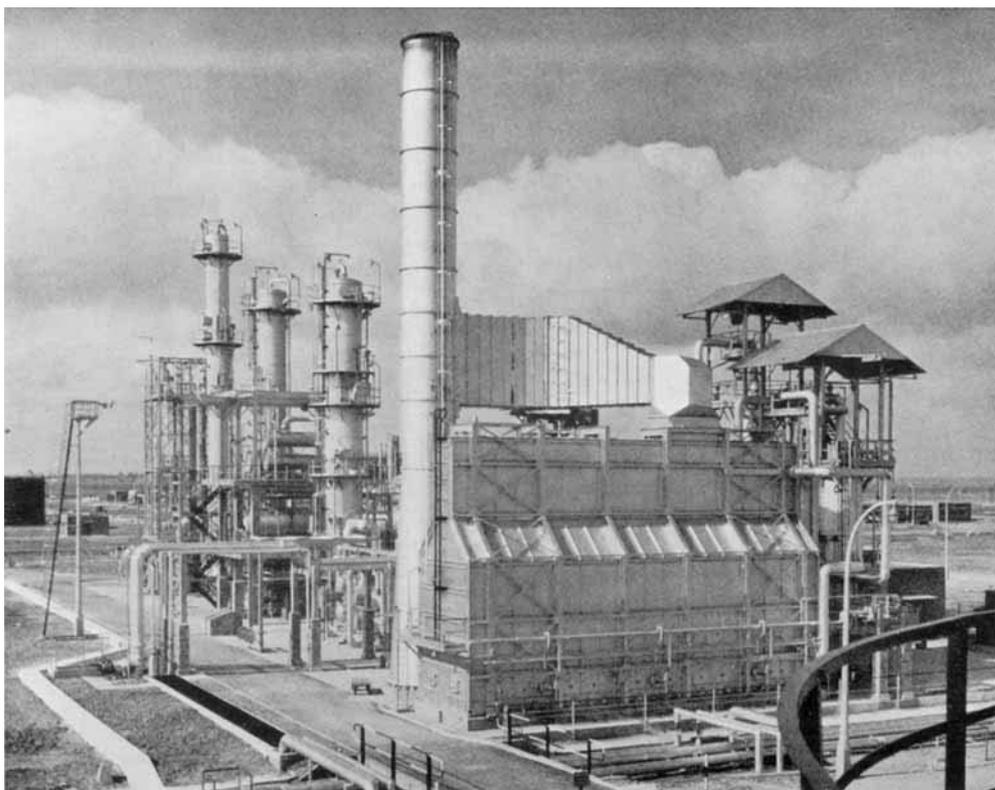
*The Platforming unit at the Kent Refinery of the British Petroleum Company Ltd. on the Isle of Grain. This has a capacity of 6,000 barrels per day*
