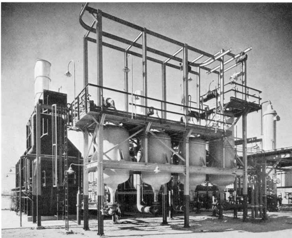
*The heart of a Platforming unit. The catalyst is contained in the four squat vessels in the foreground; the heater is on the left of the photograph*
