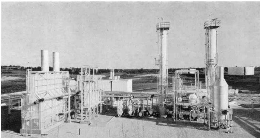
*A typical 5,000 barrels per day Platforming unit processing mid-continent naphtha*
