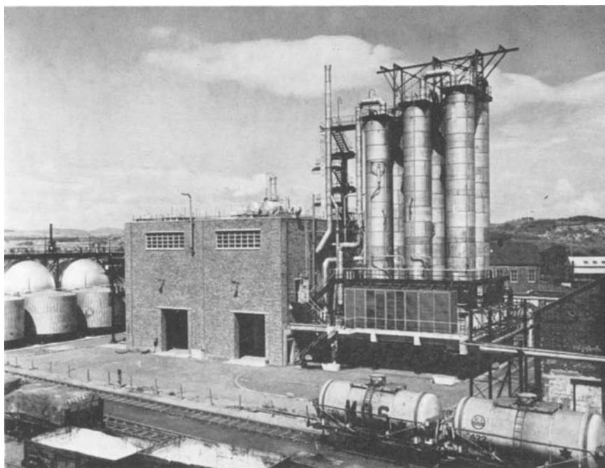
*Fig. 1 The nitric acid plant of the Nobel Division of Imperial Chemical Industries Limited at Ardeer in which the investigations on the frequency of catalyst gauze pickling were conducted. The use of the cusum method has enabled the plant to increase significantly its overall efficiency*
