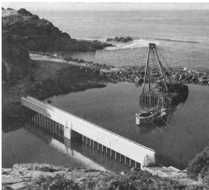
*The anode installation at the Italian mainland end of the 200 kV power link (Photograph by courtesy of The English Electric Co Ltd)*
