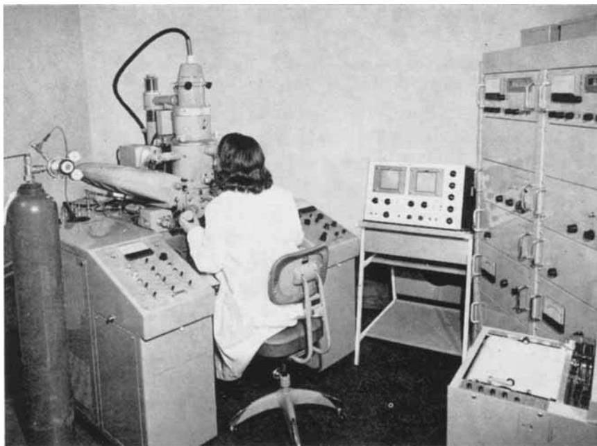
*The study of the distribution and identification of phases in an alloy system was formerly a lengthy and tedious process. The electron probe micro-analyser makes it possible to establish the structure of an alloy accurately and rapidly*
