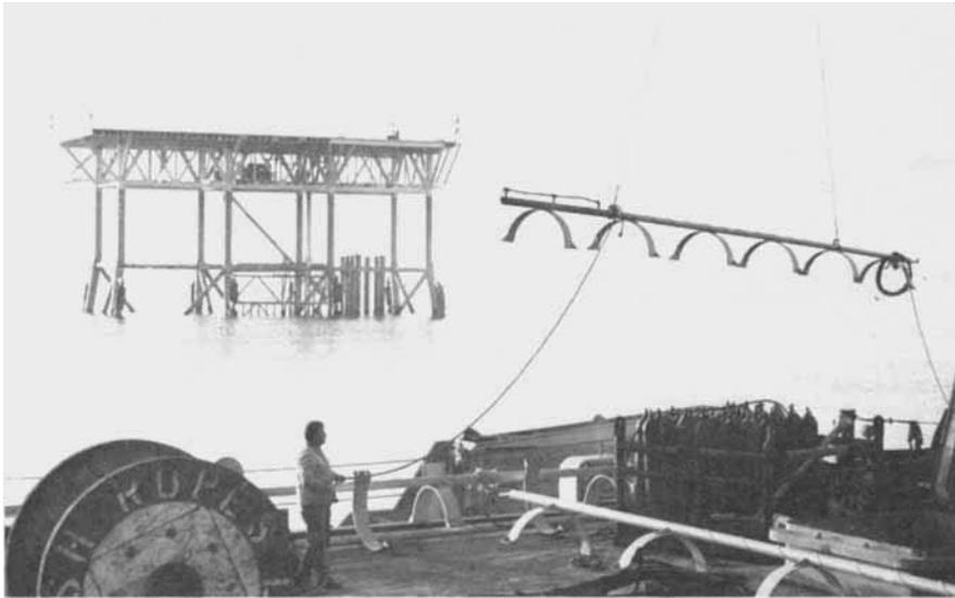
*Among the applications for which lead-platinum bielectrodes have been found successful is the cathodic protection of the structure and well casings of North Sea drilling rigs. Here an electrode - fixed at the left-hand end of the steel frame - is being installed on one such rig. This electrode will operate at 35 amps per square foot*
