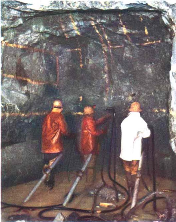
*A machine crew drilling holes for blasting in the development end of a haulage tunnel*
