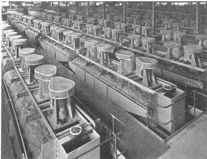
*One of the flotation plants at Rustenburg. The concentrates are thickened, filtered, dried, and pelletised before smelting to a matte*
