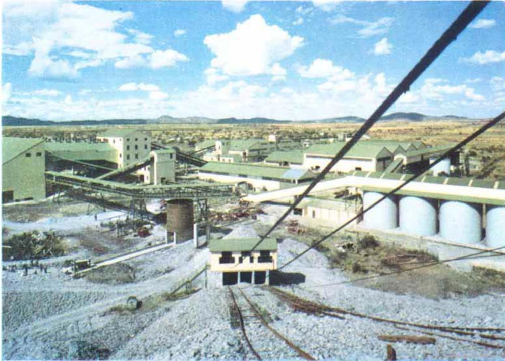
*A general view of one of the reduction plants taken from the waste rock dump. The operations carried out here include crushing the ore, milling and flotation*
