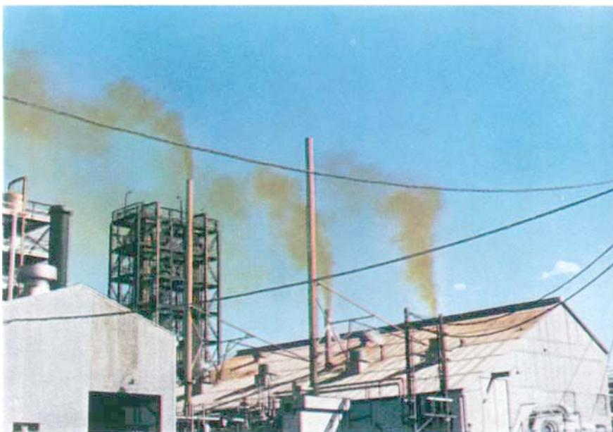
*Fig. 1 The successful use of THT platinum catalyst is seen here in a nitric acid plant. The centre stack, fitted with the catalyst system, is free from fume while the other three stacks are emitting nitrogen oxides. These three stacks have since been equipped with THT catalyst units and all are now completely clear*
