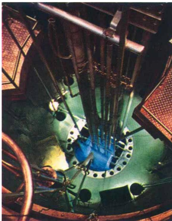
Cherenkov effect, the result of the electrons in the water becoming accelerated to speeds which are greater than the speed of light in water. On collision with other water atoms energy is released as light in the blue area of the spectrum.
