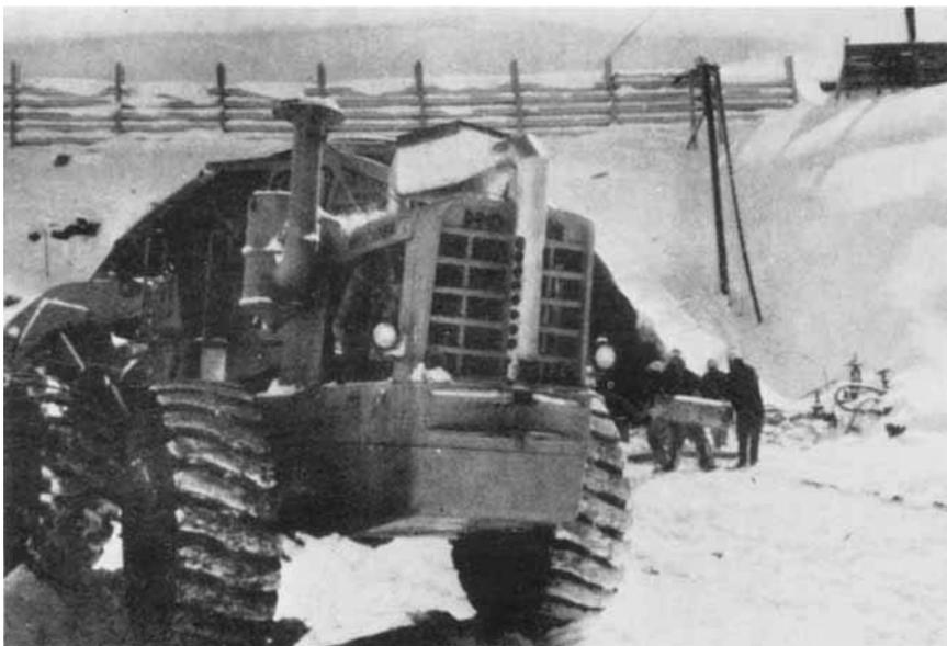
*Fig. 5 The effectiveness of the THT catalytic combustion system for diesel exhaust purification has been proved by extensive field tests. The photograph shows a large diesel tractor fitted with a THT unit to enable it to work in the Straight Creek tunnel in the Rockies*
