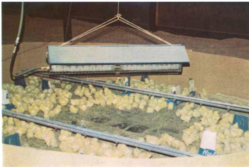
*Fig. 1 The Super-Ray propane gas catalytic heater was developed mainly for chicken brooders. Made by Impala Industries Inc. for sale to farmers by the Anderson Box Company of Indianapolis, it incorporates a tubular Cataheat flameless combustion system fabricated by Matthey Bishop Inc. This type of unit is particularly economic in fuel consumption. Although the air in the brooder pen does not feel very warm the chicks are penetrated by the infra-red radiation and hence feel comfortable*
