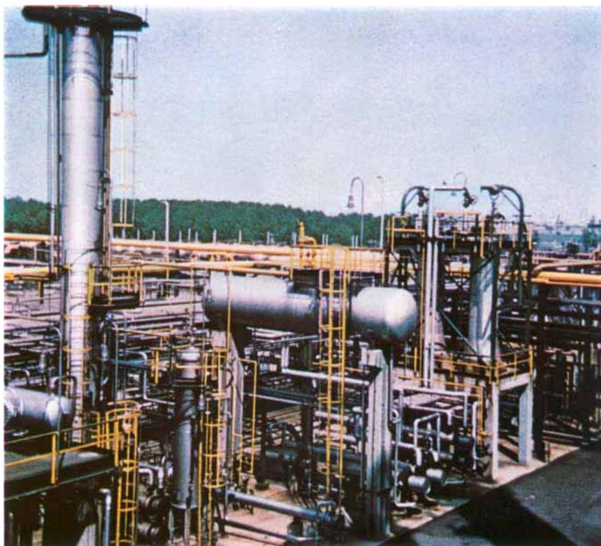
*Fig. 5 Processes are now available to isomerise paraffins to more highly branched isomers, bringing the octane number up to well over 90 RON with little or no loss of yield. This is a U.O.P. Penex unit, employing platinum catalyst on a highly acidic modified alumina support, for the isomerisation of C<sub>5</sub>/C<sub>6</sub> paraffins*
