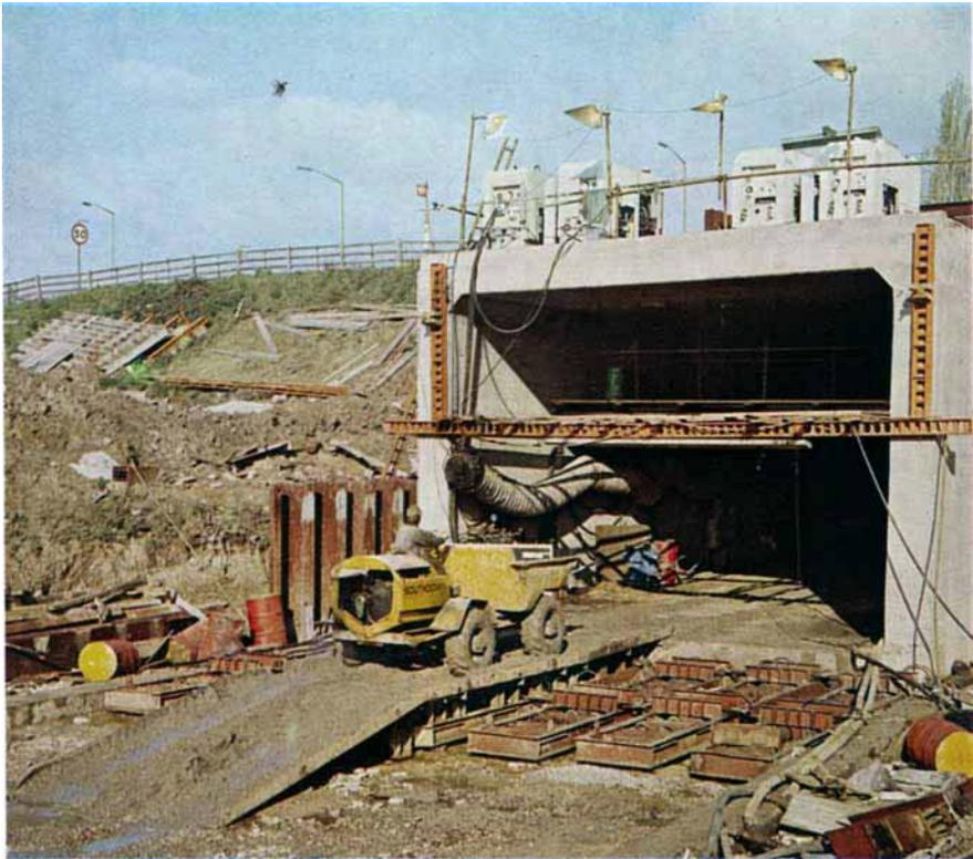
*The elimination of noxious emissions from equipment used in tunnel construction is obviously necessary to safeguard the health of those engaged in the work. This dump truck owned by Southdown Plant Limited has been fitted with a Honeycat DEP unit before use by Tube Headings Limited in driving a tunnel beneath a main road in north London*
