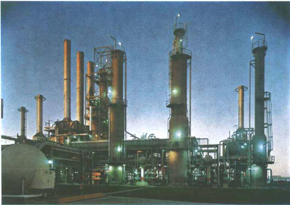
*A continuous Platforming unit in operation at the Chamlin Petroleum Company, Corpus Christi, Texas. Six such units are now on stream and a further forty-six are in various stages of design and construction*
