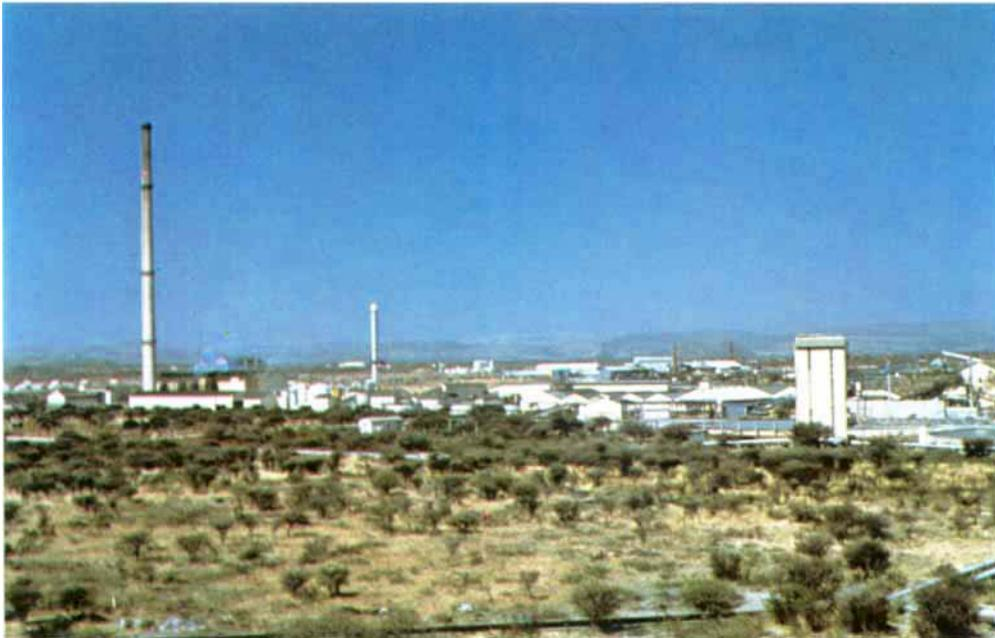
**The Waterval smelter complex shown here is one of four such plants within the company where the mineral brought to the surface is crushed, treated and smelted to a matte**
