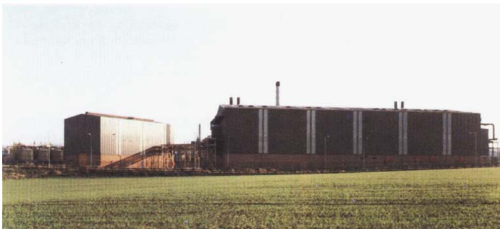
**Fig. 1** The new refinery has been built to the north of the existing facilities. The Solvex Building, shown here, houses both process facilities and support units. The process plant is divided into sections, one houses the solvent extraction equipment, another the feed preparation and interstage treatment plant; the metal refining stages are also carried out here
