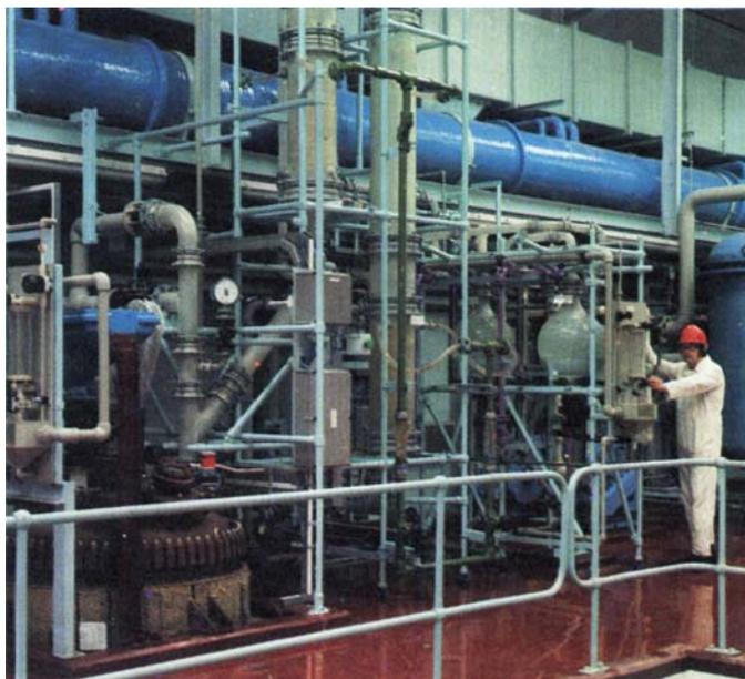
The new Royston refinery which is shown in Figure 1 has four major process areas, all of which are fully integrated. They are feed preparation, solvent extraction, metal refining and values recovery plant.
