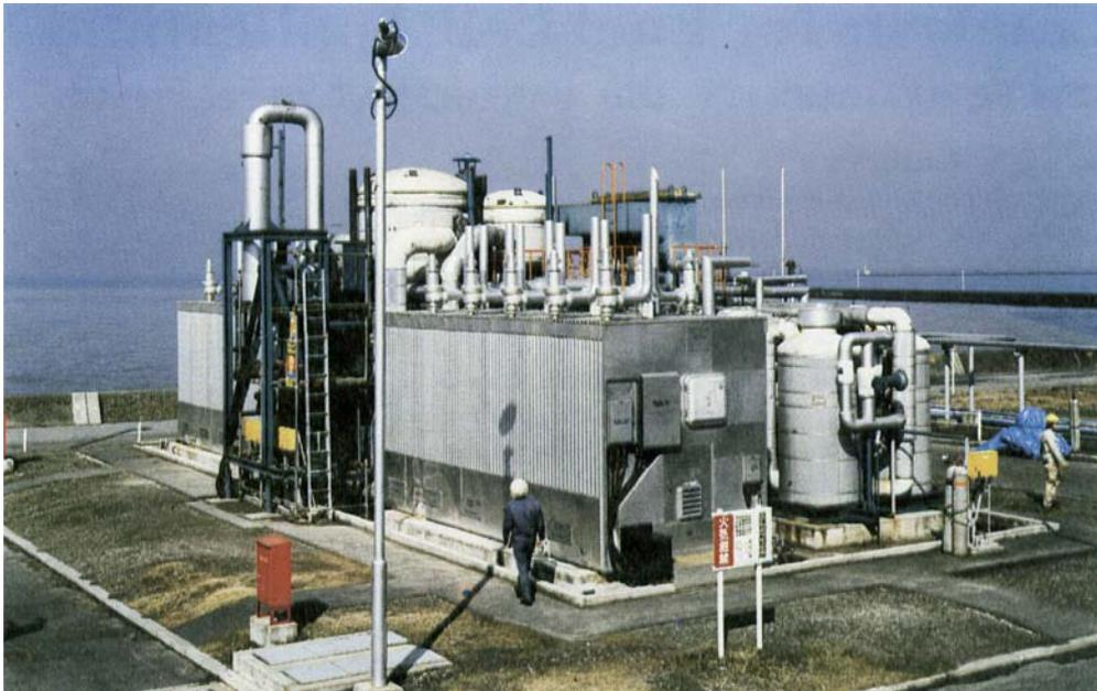
**Fig. 1** The 4.5 MW fuel cell power plant in Tokyo was constructed by United Technologies Corporation and installed by Toshiba in less than three years. Since April 1983 it has been operated at between 25 and 100 per cent of rated output. The power section, in the foreground, contains platinum catalysts supplied by Johnson Matthey
