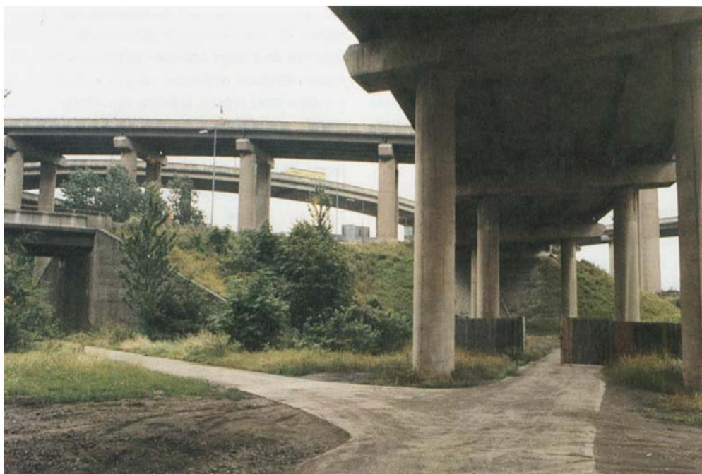
**Fig. 1 Reinforced concrete is widely used as a constructional material for structures that are required to withstand more than simple compressive forces. This section of motorway viaduct in the English Midlands is just one example of the many crucially important uses of the material**
