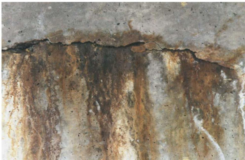
**Fig. 2 Premature deterioration of concrete can result from corrosion of the steel reinforcement bars. Commonly this is due to the action of de-icing salts on finished structures, but it may also be caused by chloride-containing setting additive or contaminated make-up water. Bulky reaction products can result in spalling of the concrete cover and mechanical weakening of the whole structure**
