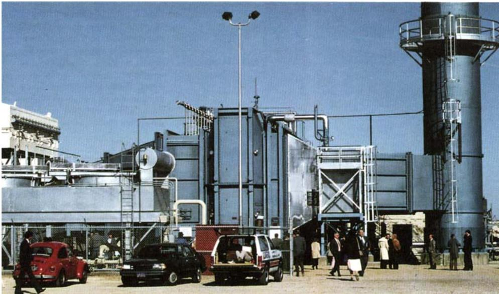
**Fig. 1** A Johnson Matthey emission control reactor is located in the centre of this picture, between the gas turbine and the stack. This reactor contains several catalyst panels measuring 10 feet by 14 feet, and purifies 4 million cubic feet of flue gas per hour. The steam from this plant is pumped underground to assist in the recovery of viscous oil
