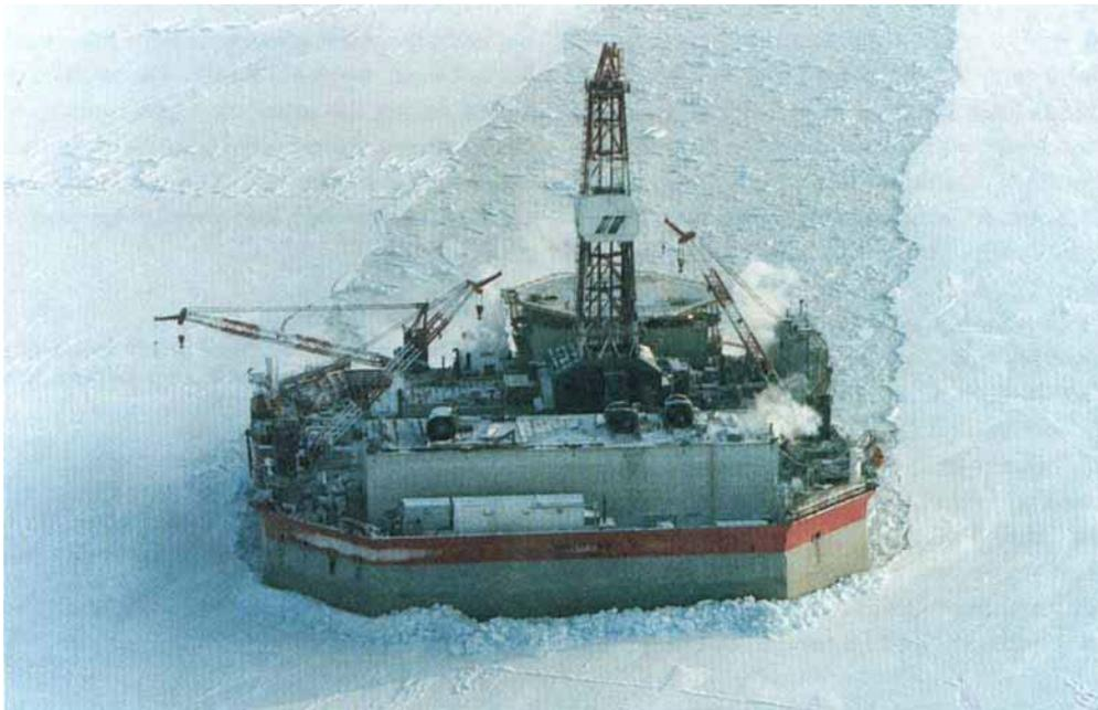
**The stationary caisson rig “Molikpaq” has horizontal loads of up to 500 pounds per square inch exerted on the hull as ice, four metres or more in thickness, attempting to flow past—due to the rotation of the earth—piles up above and below sea level. To prevent corrosion of the steel hull, twenty-four anode assemblies are employed, each of which carries two anode mounting plates which also act as primary dielectric shields**
