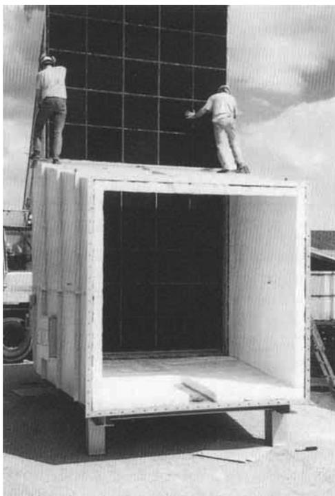
**Fig. 2** The platinum-based catalyst, supplied in the form of metal honeycomb monoliths welded together to make two large panels, is being lowered into a purpose-designed reactor housing. The catalytic reactor is fully insulated to ensure maximum temperature of the gases reaching the catalyst, in order to attain the highest oxidation performance
