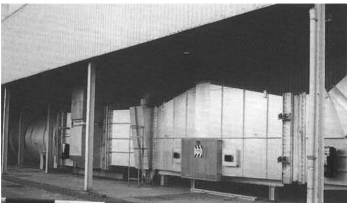
**Fig. 3** Installation of the catalytic reactor at Alcoa Manufacturing (GB), Swansea, was completed within 48 hours, requiring the minimum shutdown on the coil coating plant. As presented in a consultant's initial evaluation the catalytic reactor has shown significant savings both in capital cost and in process downtime when compared with the alternative methods for returning the thermal incinerator to compliance
