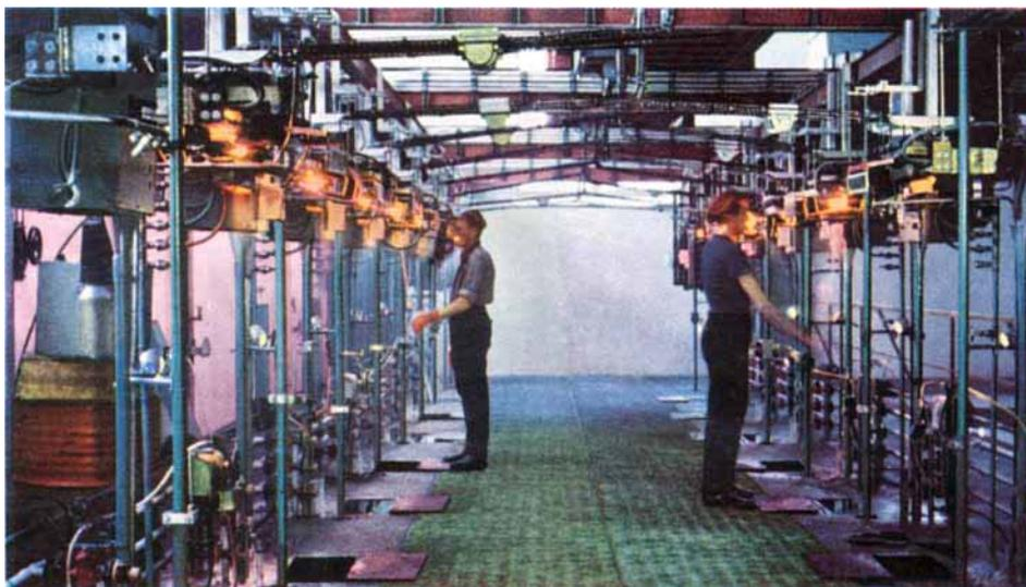
*One of the major uses of platinum in the glass industry is in the production of glass fibre in electrically heated platinum vessels or bushings. This photograph of the drawing section of the ASEA glass-fibre mill at Robertsfors, Sweden, shows the battery of bushings, operating at a temperature of around 1400°C.*
