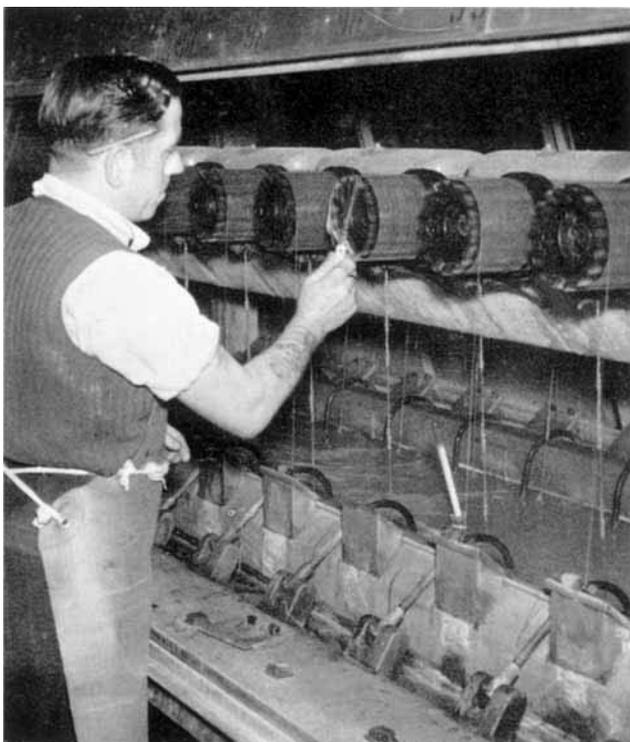
*Newly formed viscose rayon threads being led out of the coagulating bath on a textile-type continuous spinning machine in one of Courtaulds factories*
