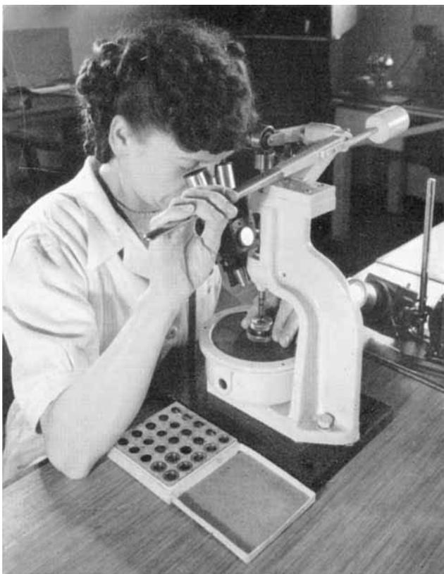
*Piercing, forming and polishing the holes in a spinning jet are intricate operations demanding considerable skill and accuracy. Here one of the operators in the Johnson Matthey jet production shop is brouching the holes in small rhodium-platinum alloy jets for spinning tyre-cord. The built-in binocular microscope is a feature of the instruments used to pierce and form the jet holes*
