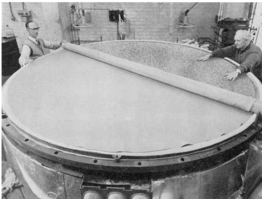
*The bottom gauze of a pad of three being placed in position in a converter. The gauzes rest on a Nimonic screen and are clamped between asbestos gaskets*
