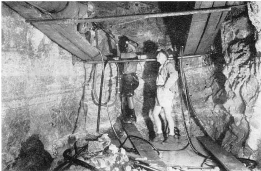
*Drilling a round of holes before blasting in a reef drive at Rustenburg*
