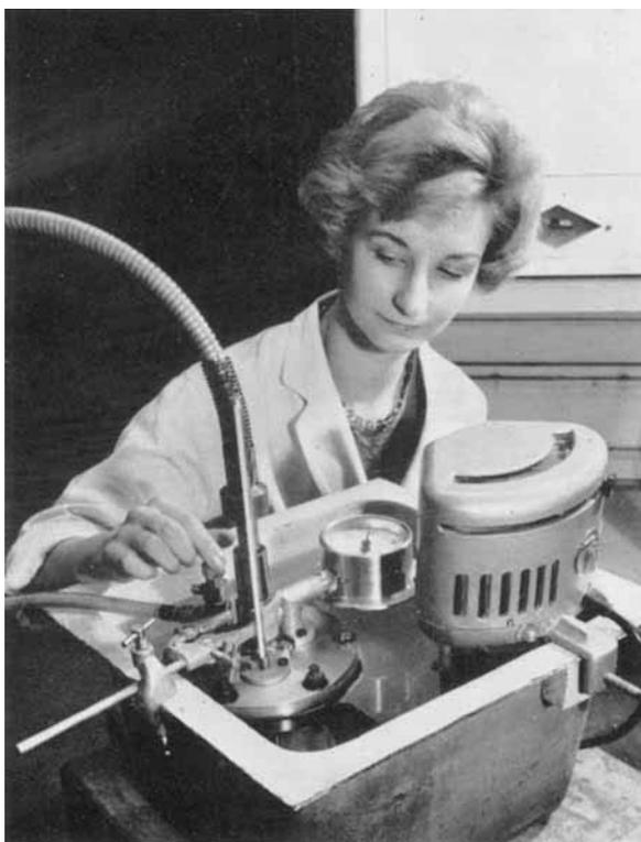
*A constant temperature autoclave for the investigation of hydrogenation reactions over charcoal-base catalysts at elevated temperatures and pressures*
