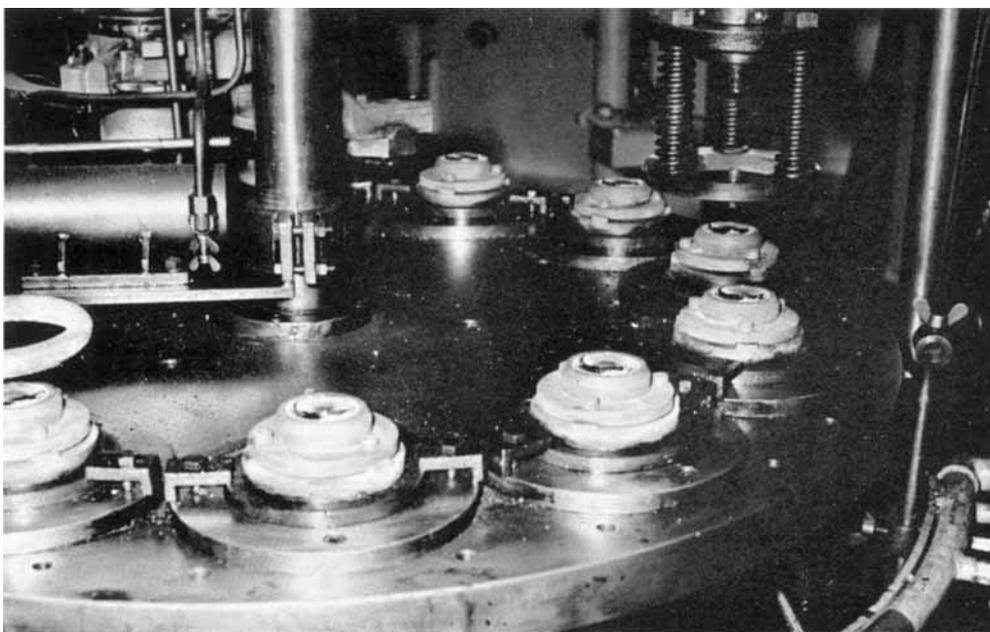
*An automatic machine in the Jena Glassworks at Mainz for the manufacture of lens blanks direct from the platinum furnace*
