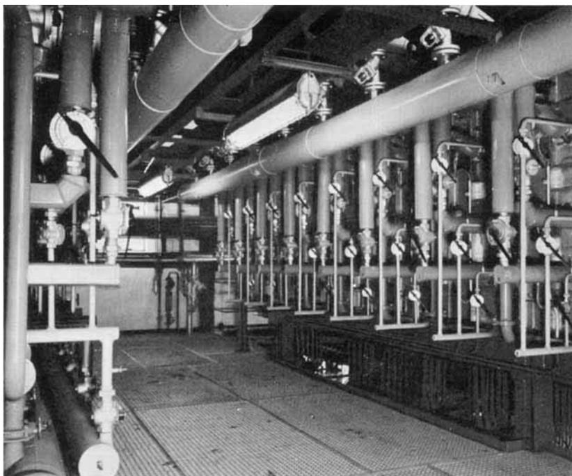
*A reactor unit producing 50 tons a month of hydrogen cyanide. Eight combustion chambers each contain thirteen ceramic tubes in which methane and ammonia react in the presence of a platinum catalyst*
