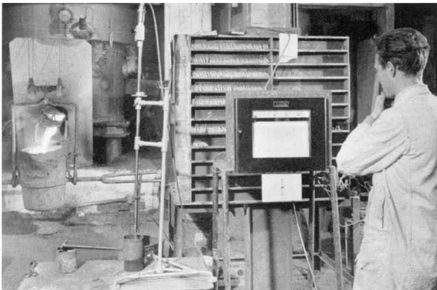
*The BCIRA method in use in an automobile foundry, with a Honeywell temperature recorder directly calibrated in terms of the carbon equivalent. Results can be obtained in less than two minutes before castings are poured, so that corrective measures can be taken rapidly. The pyrometer and stand were designed by Amalgams Limited*
