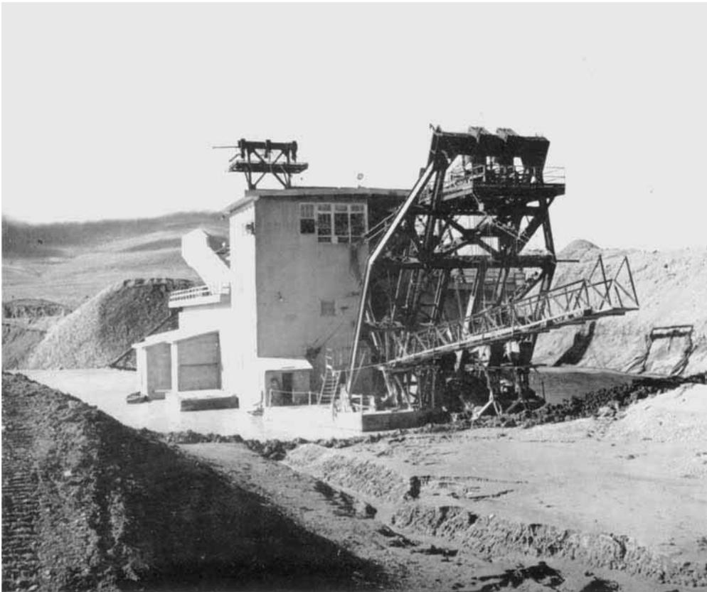
*The digging ladder of the dredge carries a line of ninety-four buckets, each of eight-cubic-feet capacity. The dredge is capable of digging fifty feet below water level to reach the platinum-bearing gravel*
