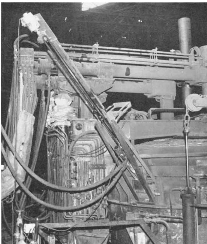
*The water-cooled probe installed in an arc furnace. Entry and withdrawal, governed by electric motor, are effected through a 5-inch diameter hole pre-cast in one of the dolomite blocks used for lining the side wall of the furnace*
