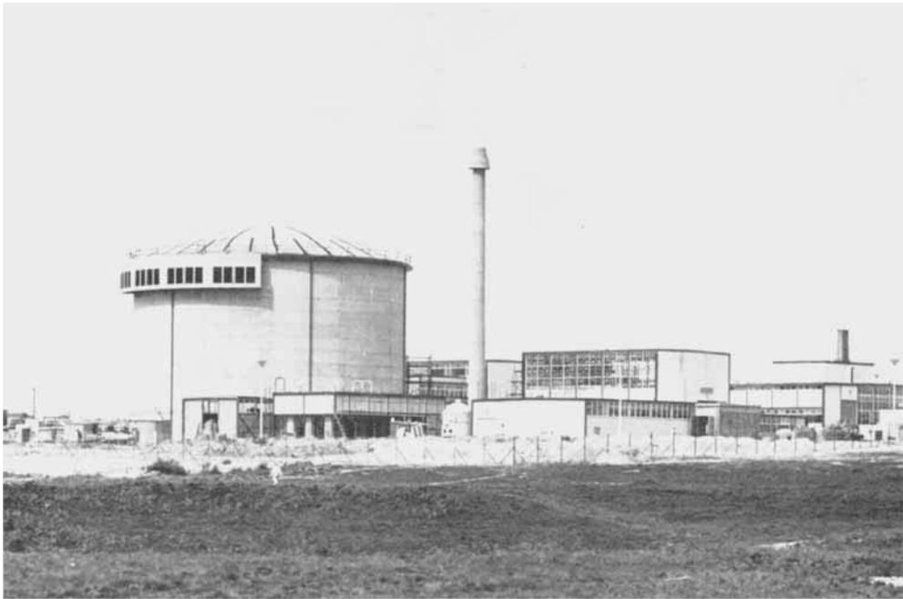
*The Dragon Reactor – the high temperature gas-cooled reactor experiment – is being built by twelve European countries, all members of the Organisation for Economic Co-operation and Development (OECD). One of the main objects is to gain operating experience with graphite uranium carbide fuel elements operating at high temperatures for prolonged periods. The outlet temperature of the helium coolant permits steam to be produced with characteristics suitable for modern turbo-alternators*
