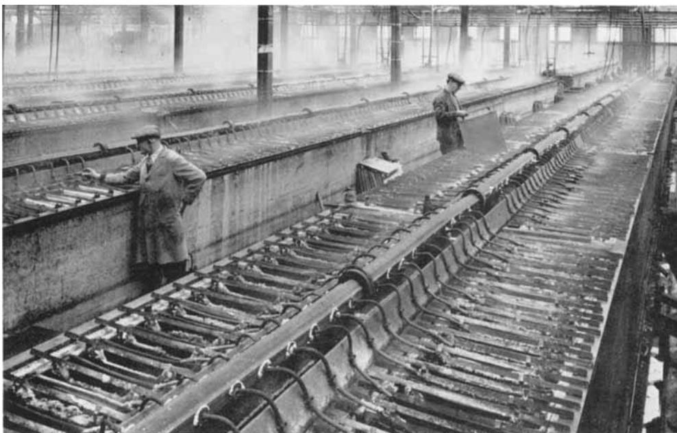
*The electrolytic nickel refinery at Brimsdown. Here pure nickel cathodes are produced, while the platinum metals accumulate in the anode residues and are removed for the separation and refining of the individual metals*
