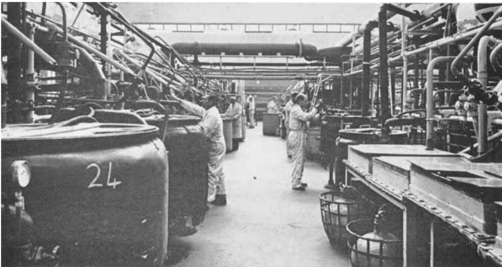
*In this part of the refinery the four “insoluble” metals – ruthenium, rhodium, iridium and osmium – are extracted and separated as their complex ammonium salts*
