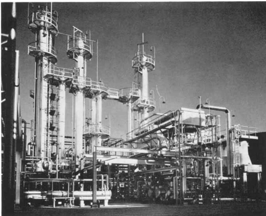
*A Hydrar process unit at an Oklahoma refinery. A platinum catalyst is used for the conversion of benzene to high purity cyclohexane, mainly for subsequent oxidation to adipic acid in the preparation of Nylon-type polyamides*
