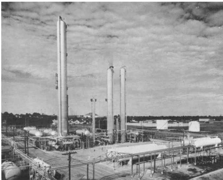
*The Penex process employs a platinum catalyst specifically designed for the hydroisomerisation of pentanes and hexanes to highly branched isomers for use in high octane fuels. This Penex unit forms part of a refinery in Louisiana*
