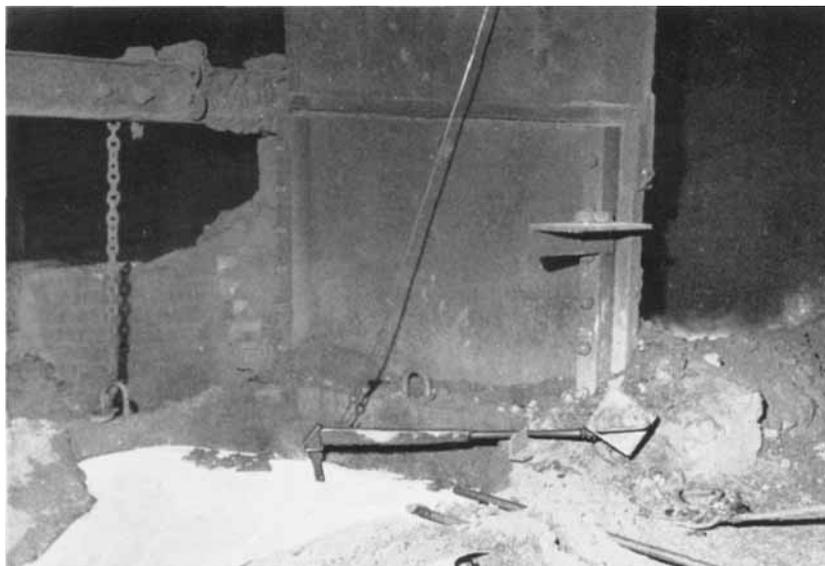
*The Gee continuous immersion thermocouple in position in the stream of molten iron flowing from a blast furnace in one of the Bethlehem Steel Company's plants*
